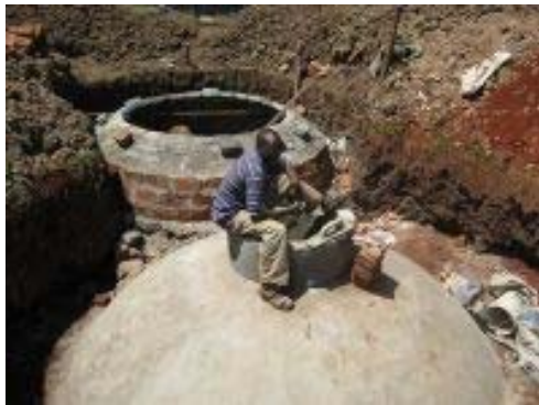
Construction of an Ikotoilet (Photo credit: Ecotact)
