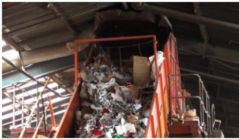
Mondi recovery facility – (Photo credit: Pierre Coetzer)
